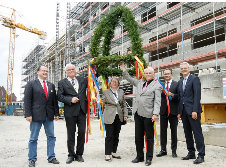
A topping-out garland for the BRICS. From left to right: Prof. Dieter Jahn, Vice President of the TU Braunschweig, Prof. Jürgen Hesselbach, President of the TU Braunschweig, Renate Müller-Steinweg, supervisor of the Staatliches Baumanagement Braunschweig (Department of building inspection), Peter-Jürgen Schneider, Minister of Finance of the state of Lower Saxony, Ulrich Markurth, Mayor of Braunschweig, Prof. Dirk Heinz, Scientific Director of the HZI. Photograph: TU Braunschweig/Presse und Kommunikation
